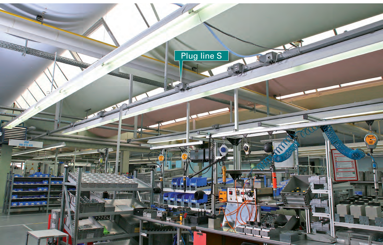
At Dungs in Urbach, the plug line S was mounted to square pipes (80 mm), which serve as compressed air piping and storage at the same time.
