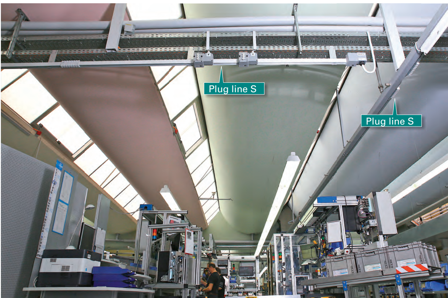
At Dungs in Urbach, the plug line S was mounted to square pipes (80 mm), which serve as compressed air piping and storage at the same time.
